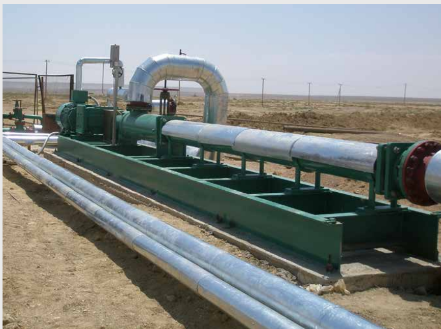
NM090SY Capacity: 11,5-50-55 m 3 /h Pressure: 23-30-35 bar Medium: oil, water, gas Gas rate: 35%
